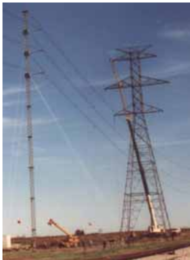
Three Phase Running Angle: This 30 degree 500kV ERS was built to restore power after the permanent tension tower was sabotaged.
