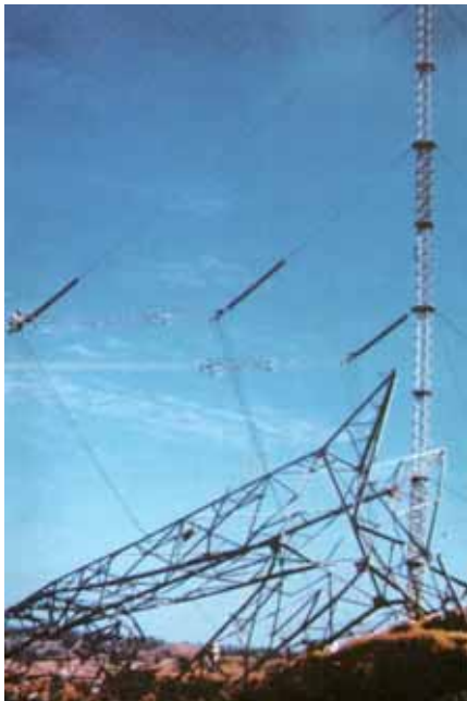
DC Chainette: This +/-500kV Direct Current ERS was built in One day when an airplane destroyed the permanent tower.
