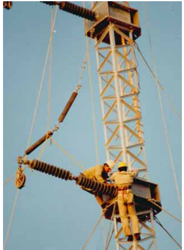
Above, the 7155 Box Section is used to support the post insulator used in a typical Horizontal-Vee ERS Structure.
