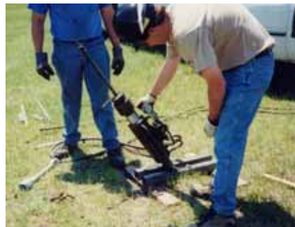
Left to right: Starting to install, installing and final locking of the normal soil density hydraulically installed self locking anchor. A Complete anchor installation kit is shown above right.
