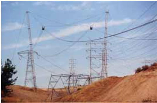
DC Chainette: This +/-500kV Direct Current ERS was built in One day when an airplane destroyed the permanent tower.
