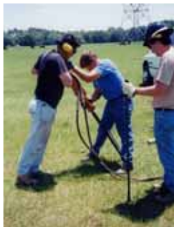
Left to right: Starting to install, installing and final locking of the normal soil density hydraulically installed self locking anchor. A Complete anchor installation kit is shown above right.
