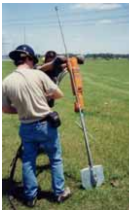
Left to right: Starting to install, installing and final locking of the normal soil density hydraulically installed self locking anchor. A Complete anchor installation kit is shown above right.
