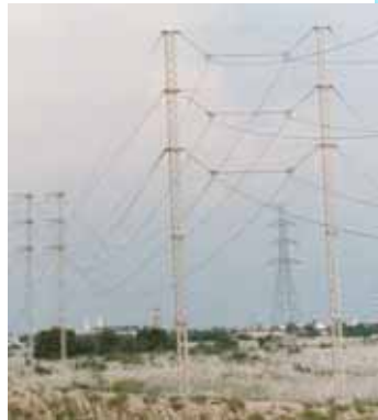
Double Circuit Herringbone: This Double Circuit 230kV ERS was built after a major disaster. The picture at the left shows the same ERS still in service 8 years later.
