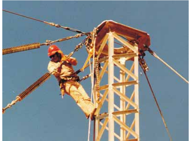
Part No. 7157 45°/45° Guy Plate, shown above, can be located at the top of columns or placed between column sections.
