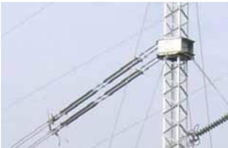
Left, a 7155 Box Section is used to provide vertical bundle separation of a 4-conductor per phase Tension ERS Structure.
