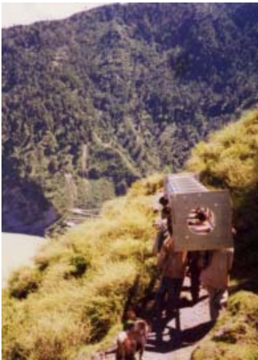
Figure 2 Fourteen-foot ERS column section being hand carried to the construction site, along a typical trail.
