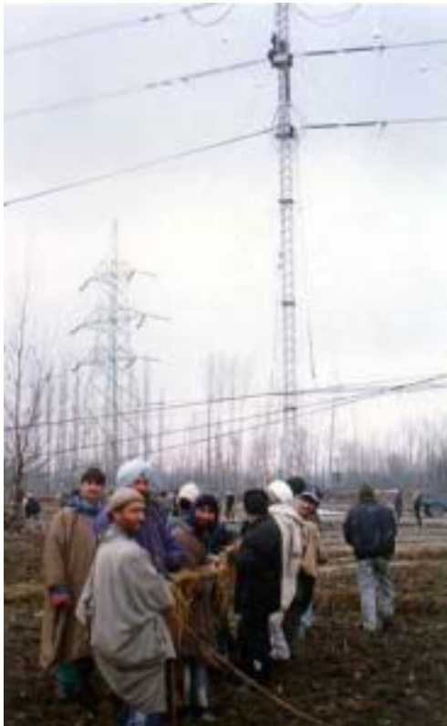
Figure 8 Erection of the 400kV single circuit 15-degree tension ERS tower using manpower to pull the two conductors of the bottom phase.
