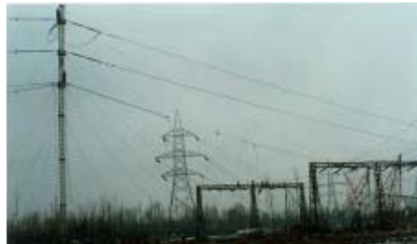
Figure 9 Two views of the almost completed 400kV ERS tension tower showing the span over the double circuit 220kV line.
