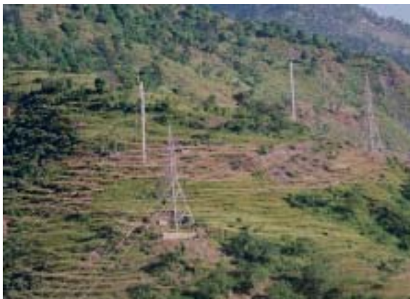
Figure 4 Completed ERS bypass of towers 58 and 59.
