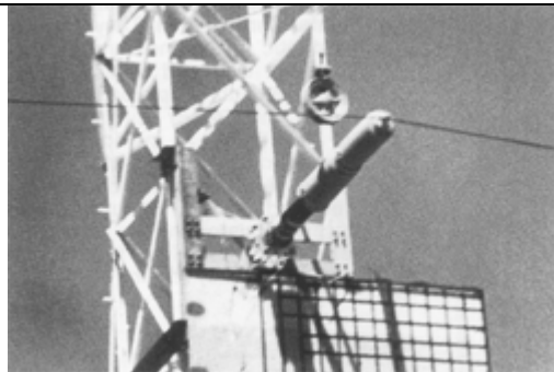
Figure 4. Tower No. 1 before test.
