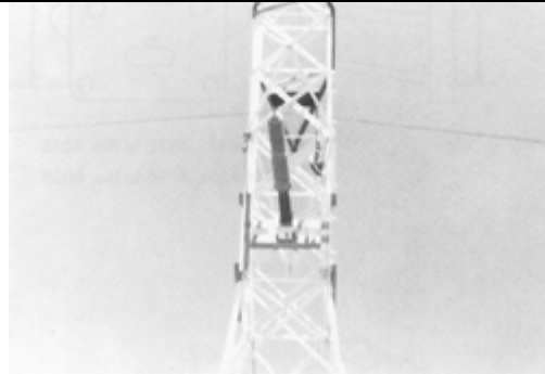
Figure 7. Tower No. 3 after test.
